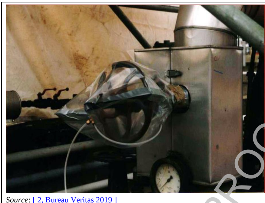
Figure 3.66: Bagging of a leaking valve
